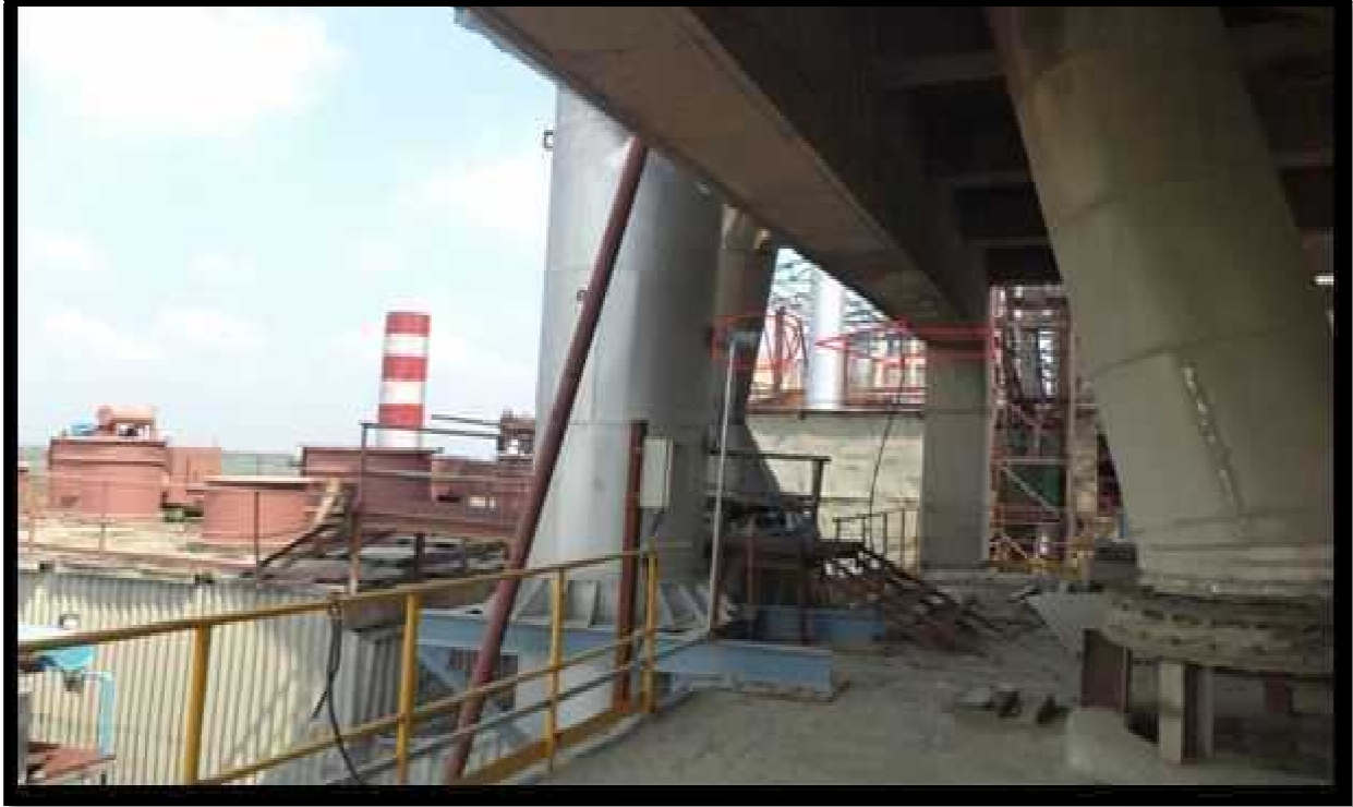
Continuous Emission monitoring Analyzer on Cement mill-1
