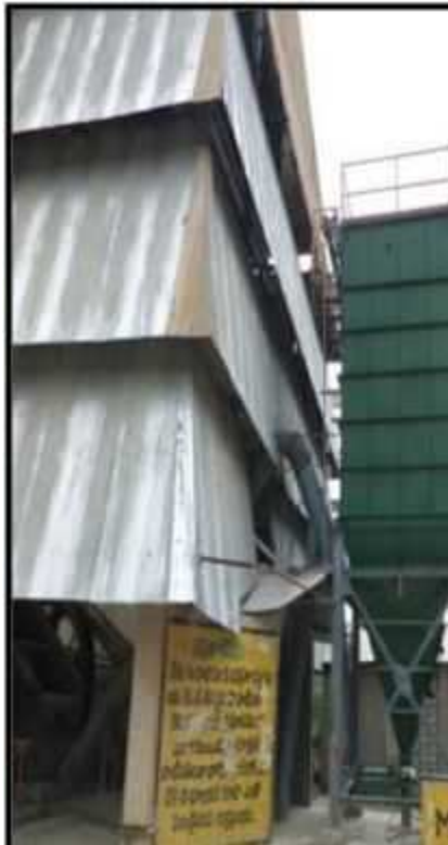
Bag Filter Installed on Crusher Bag Filter Installed in kiln feed section
