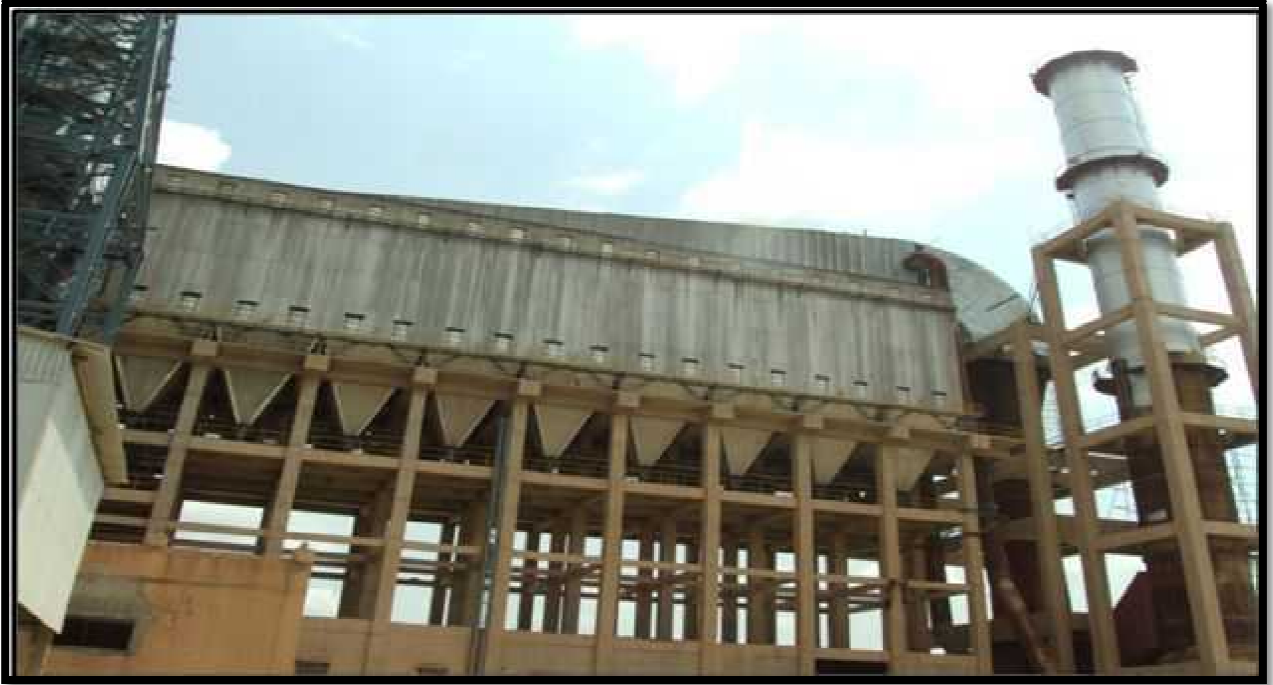
Reverse Air Bag House (RABH) Installed in Kiln & Raw millsection
